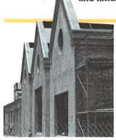
To complete the Main Church at Mary's Shrine, construction crews will use some 812,000 lbs. of structural steel, 265,000 lbs. of reinforcing steel, and more than 14 million lbs.of concrete.
