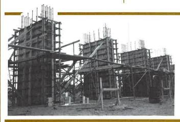
When completed, these 23-foot pillars will act as buttresses, providing support for the walls and roof of Mary's Church.
